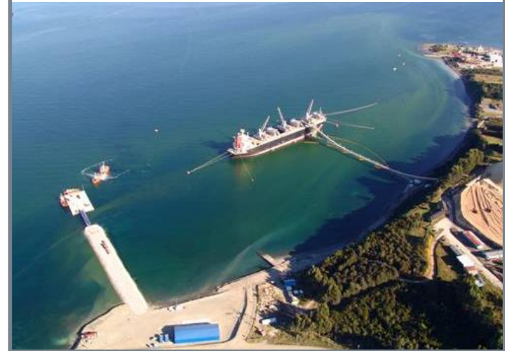
Calbuco (X Region) San Jose Dock and General Cargo Terminal
